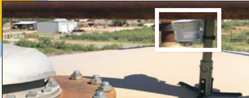
MethaneTrack™ endpoint mounted on tank near thief hatch
